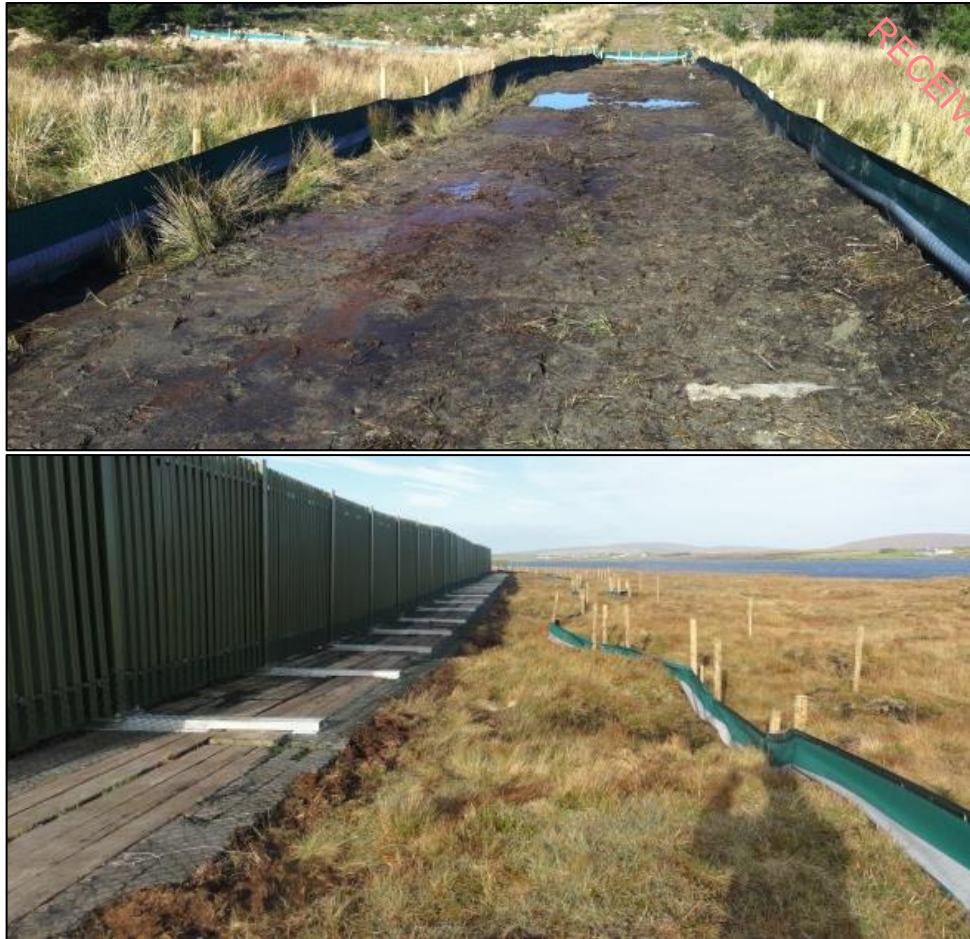
Plate 2-4 Typical Silt Fence Details
